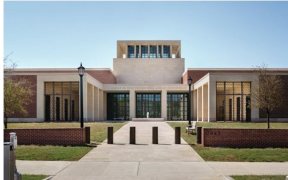
G.W. Bush Presidential Library, Robert A.M. Stern Architects LEED Platinum, 2013
