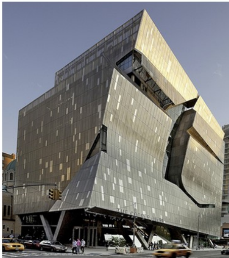
41 Cooper Square, Morphosis LEED Platinum, 2009
