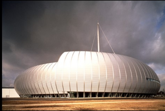
LIMOGES CONCERT HALL Bernard Tschumi Architects
